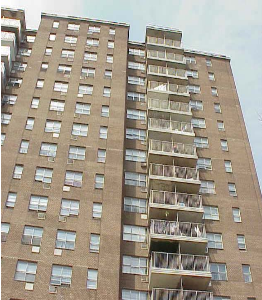
Hazel Towers 2-60 KW IC units
