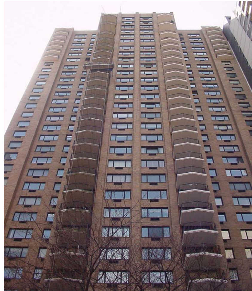
Park Ten 1-70 KW Microturbine
