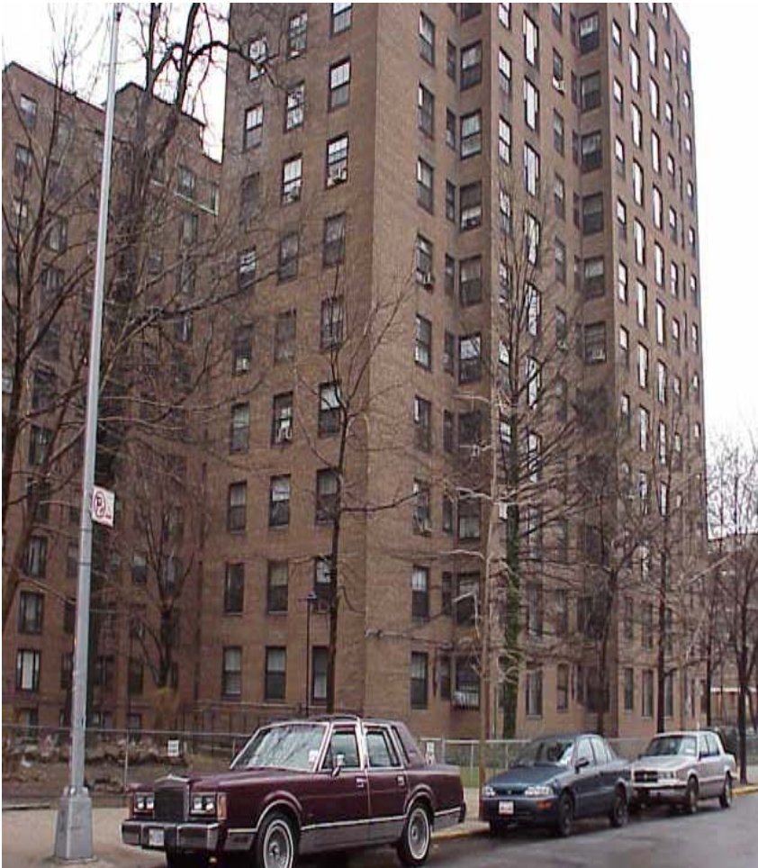
Clinton Hill Apartments Group of Microturbines
